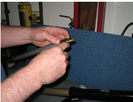
Inset the o-ring into the bottom groove
